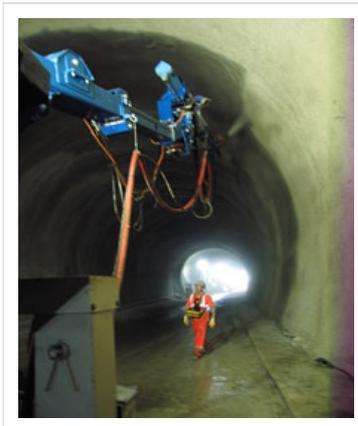
**Spray-on waterproofing as part of a composite shotcrete lining**
