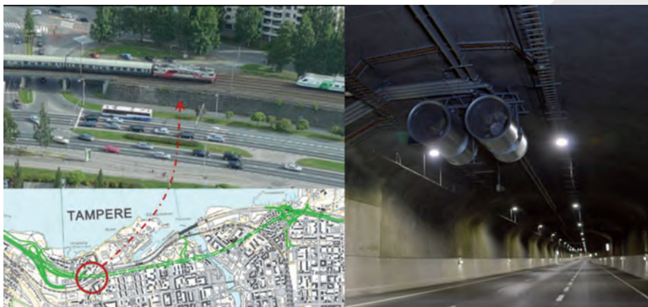
Figure 3 : An example of critical and challenging estimate of allowed vibration level. The structure of an old railroad basement was not exactly known. A crossing twin tube traffic tunnel was excavated using drill-and-blast method by Lemminkäinen Oy. Photo courtesy of city of Tampere.
