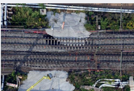
Collapse of the TBM rail link under the mainline railway at Rastatt, Germany, 2017
