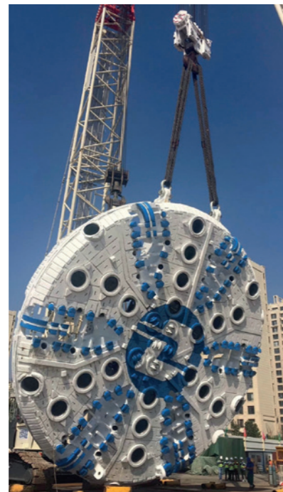
Assembly of the 12.26m cutterhead
