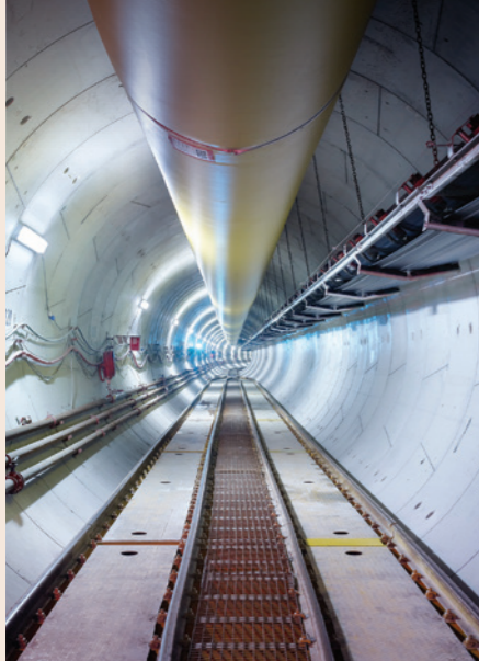
High quality finish for STEP wastewater network, Abu Dhabi, UAE, 2012
