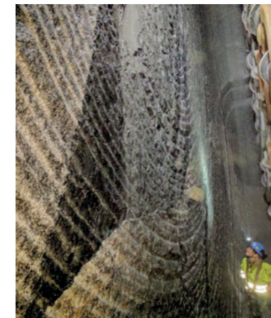
Mapping a TBM rock face
