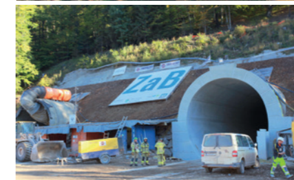
Railway tunnel portals
