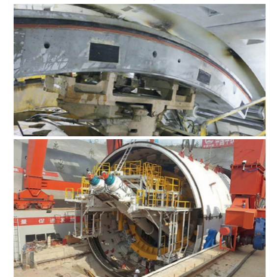
Segmental lining and mechanical erector; Double screw conveyors
