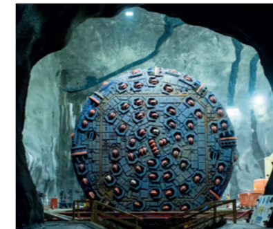
First of four TBMs ready for launch (Photo by Acciona/Ghella JV)
