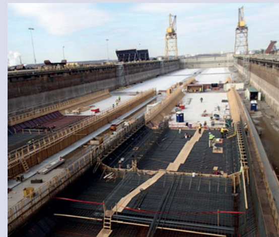
Midtown immersed tube crossing of Chesapeake Bay, USA, 2011
