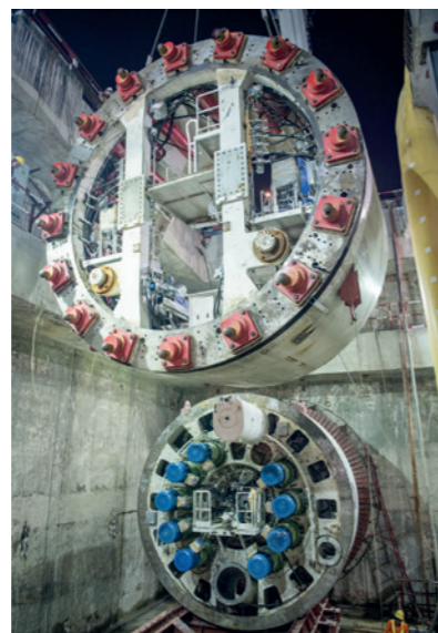
Terratec 6.39m diameter EPBM
