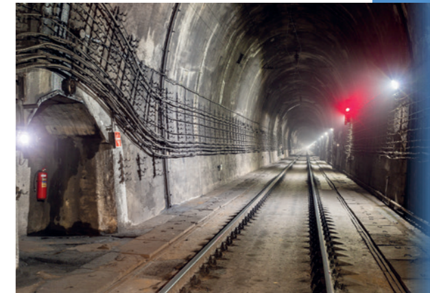
Existing single-tube, single-track, bi-directional Severomuiski tunnel
