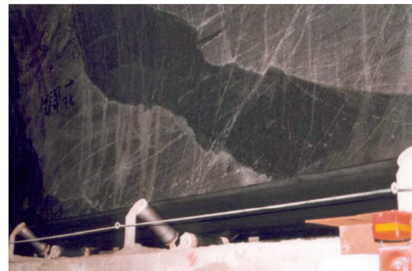
Mixed face intrusion in a hard rock mass
