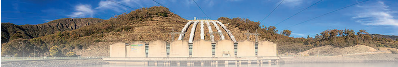
Talbingo power station and the reservoir that is to become the lower basin of the Snowy 2.0 scheme
