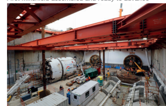
First Mixshield assembled and ready to advance
