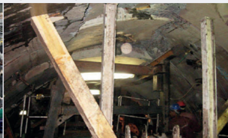
Failure of the operating headrace on the Gilgel Gibe II hydro scheme in Ethiopia, 2010
