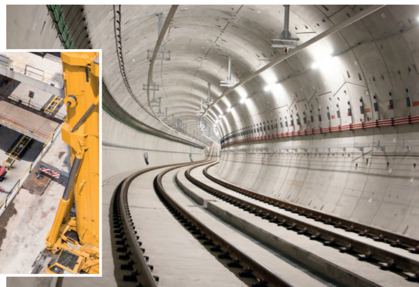
Right: Top quality single-tube, double-track metro alignment; Below: First of three EPBMs in assembly
