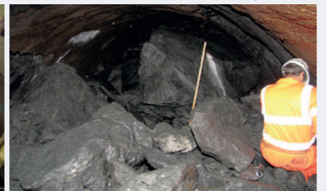
Headrace collapse after commissioning of the Glendoe scheme in Scotland, 2009
