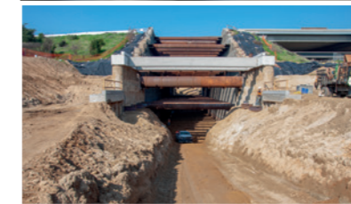
State Route 180 Fresno Trench underpass
