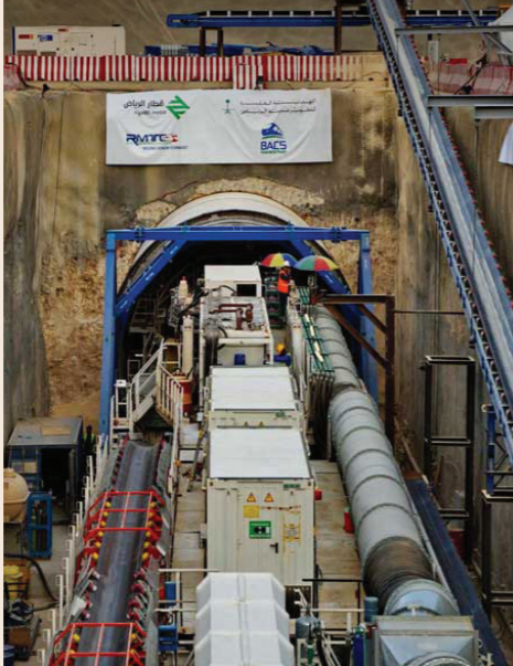
Excellent TBM performances linked metro stations in Doha, 2016
