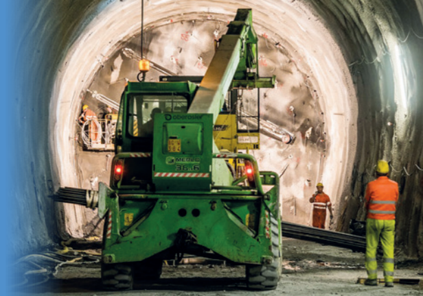
Drill+blast established start of the Mules Lot
