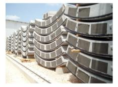
TunnelFlex 33 Plus, Rubber gaskets with 90° Soft corners
